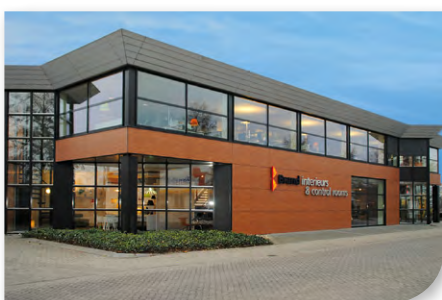
▲ Brand interiors and Brand control rooms in Deventer, NL
